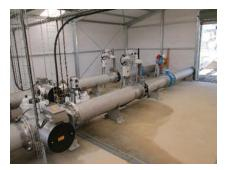
Wastewater Treatment Plant Bulk Lime Silo project has replaced the lime dosing hopper and dosing system, pipework is installed and SCADA integration complete. Dosing will minimising potential health and safety issue.
